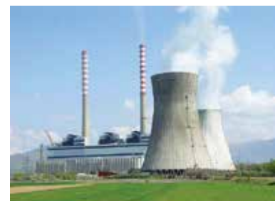
A Thermal Power Station
