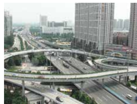
Road Network with flyovers
